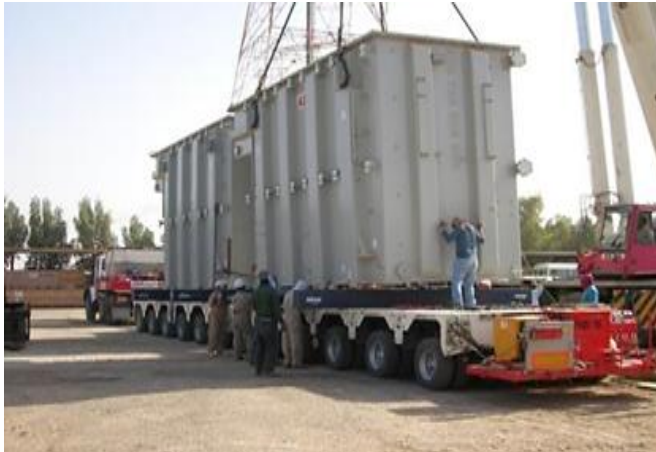
Discharged In Kuwait - Jacking & Skidding Transformers For Abb Projects
