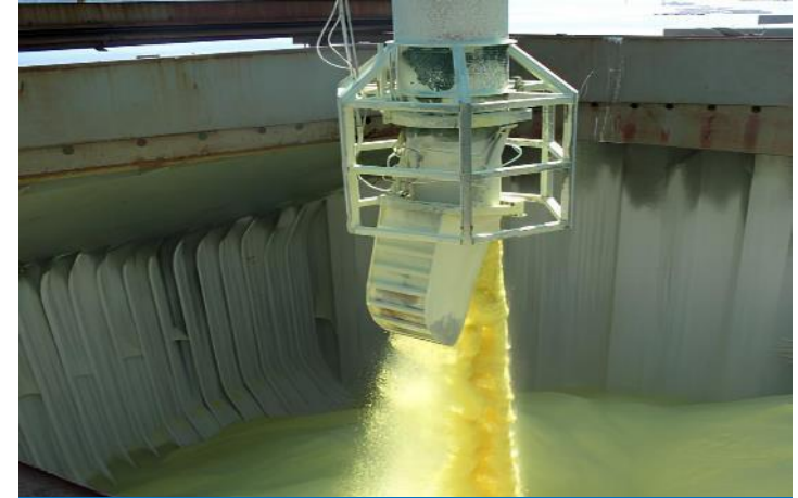
Sulphur Loading Ruwais
